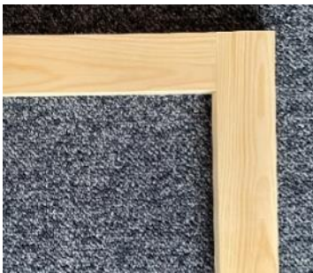
Traditional frame flush joints square inner & outer edge
